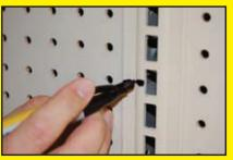
Always begin installation with the bottommost Merchandiser. Put a mark at the 5<sup>th</sup> slot from the lowest point in the plan-o-gram set. This denotes the slot into which the top tooth of the Merchandiser will be inserted.
